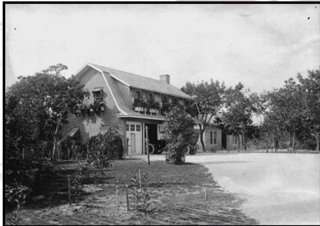
Carriage House and Power House, 1916. Photo by J.K Small
